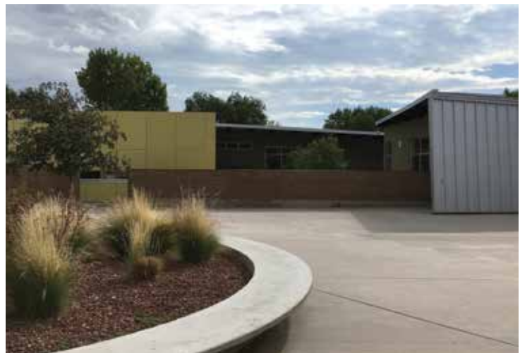
MRGC developed a partnership with APS to build their new school buildings. Through this arrangement, APS made MRGC part of their overall facilities master plan.
